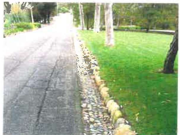
Cobble curb and gutter, 2004
